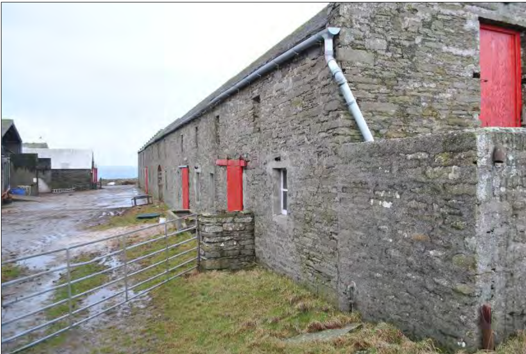
Plate 84: The south-facing elevation of Building 6.1, looking east, with the doorway providing access to the first floor grain loft visible in the top right corner.
