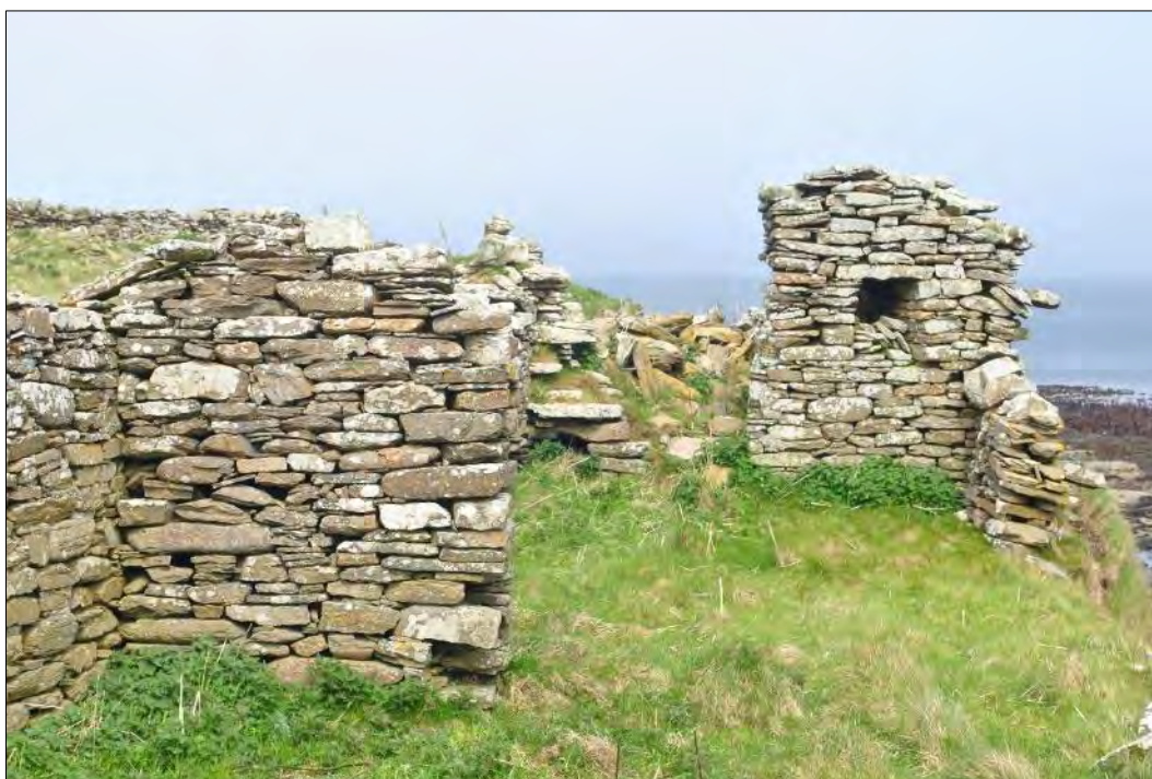
Plate 114: View from FB 2 of FB, looking northeast, showing loss of the east wall (right) and the upstanding remains of a corn drying-kiln (background centre and right).
