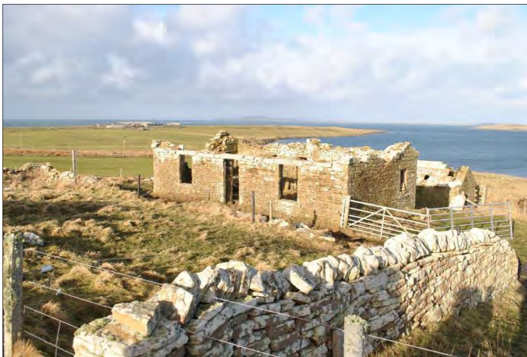
Plate 173: General view of Quarryhouse looking northwest from Westside Road. This view shows the main domestic building (Building 1), now roofless, with a later outbuilding (Building 6) behind.
