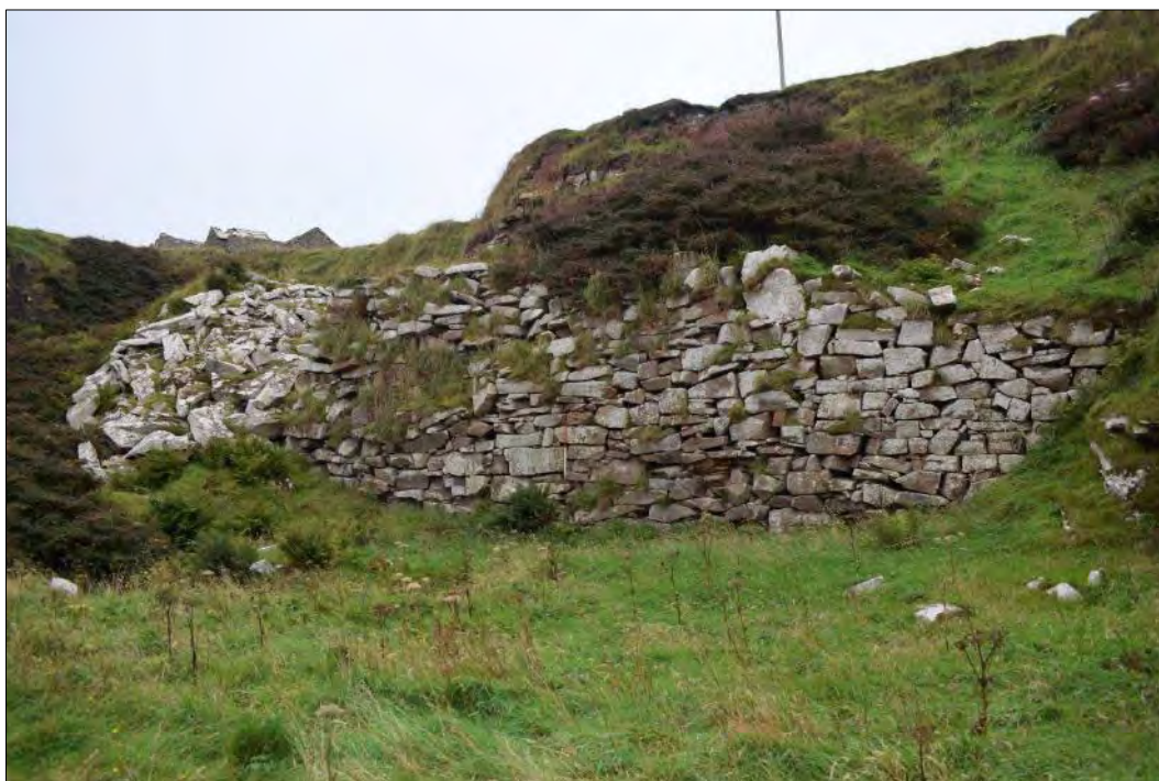
Plate 170: View from the centre of Fersness Quarry, looking towards the southwest corner, showing a pile of stone debris alongside one of the retaining walls ( Feature 20 ) constructed within the quarry.
