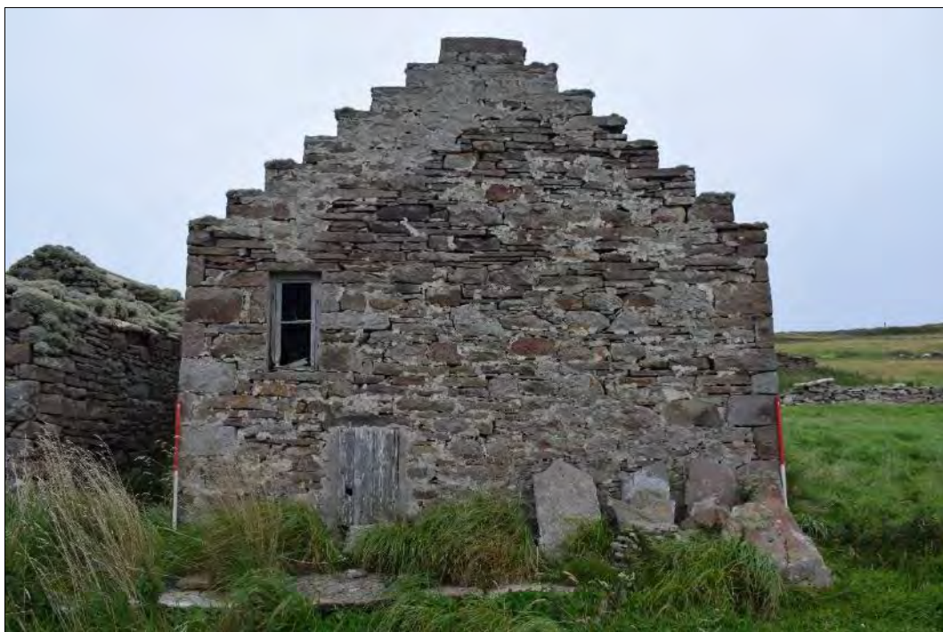
Plate 35: Crow-stepped, west-facing gable of Building 11 with small, narrow window and the oddle hole below.
