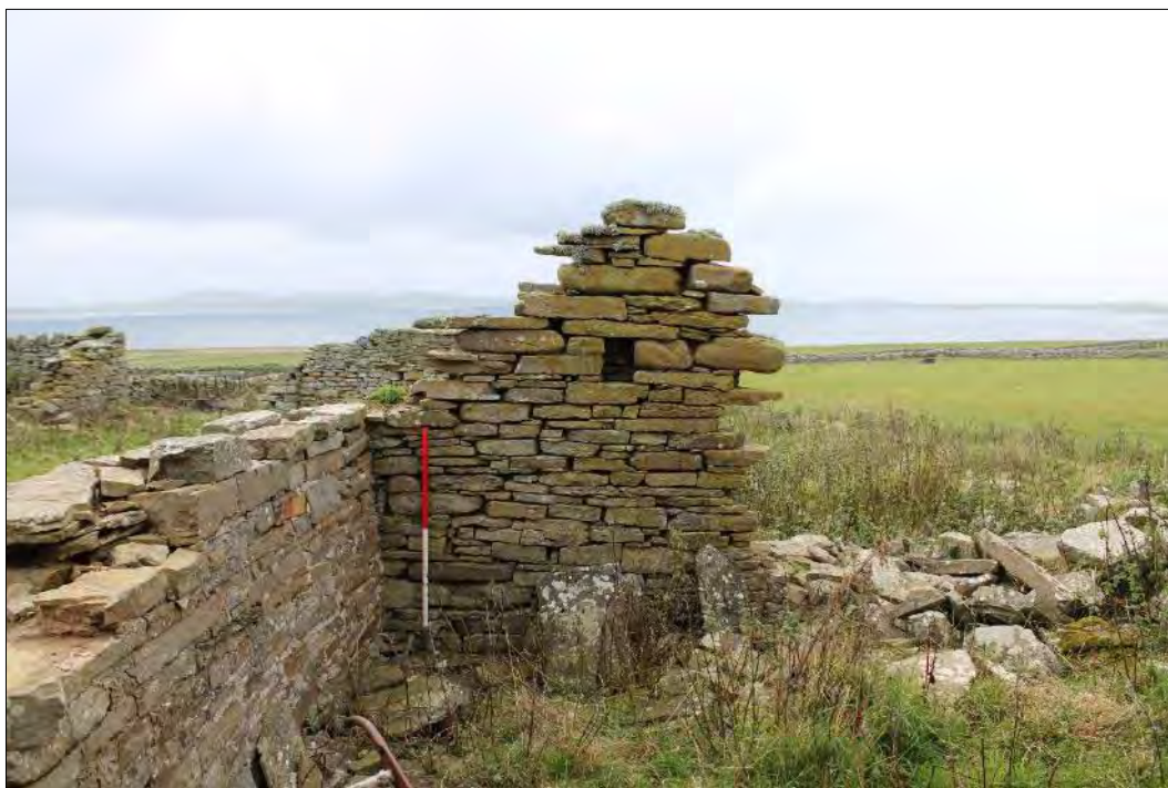
Plate 102: The east-facing gable of Building 12 with the south wall of Building 12.1 (left) butting against it. Behind the gable, to the left, is the enclosure wall between Building 12 and Building 11 and, on the extreme left, is the northwest corner of Building 11.
