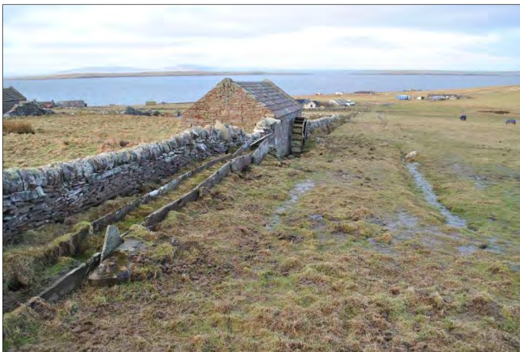
Plate 42: General view of the water-powered mill (Building 17), looking southwest, showing the canalised head race (left) and the ditch forming the tail race beyond the water wheel.
