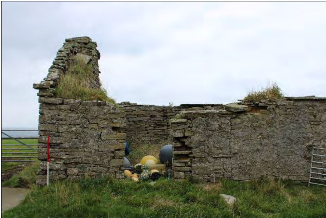
Plate 106: South-facing elevation of Building 13 showing the external doorway with the blocked window to the right.
