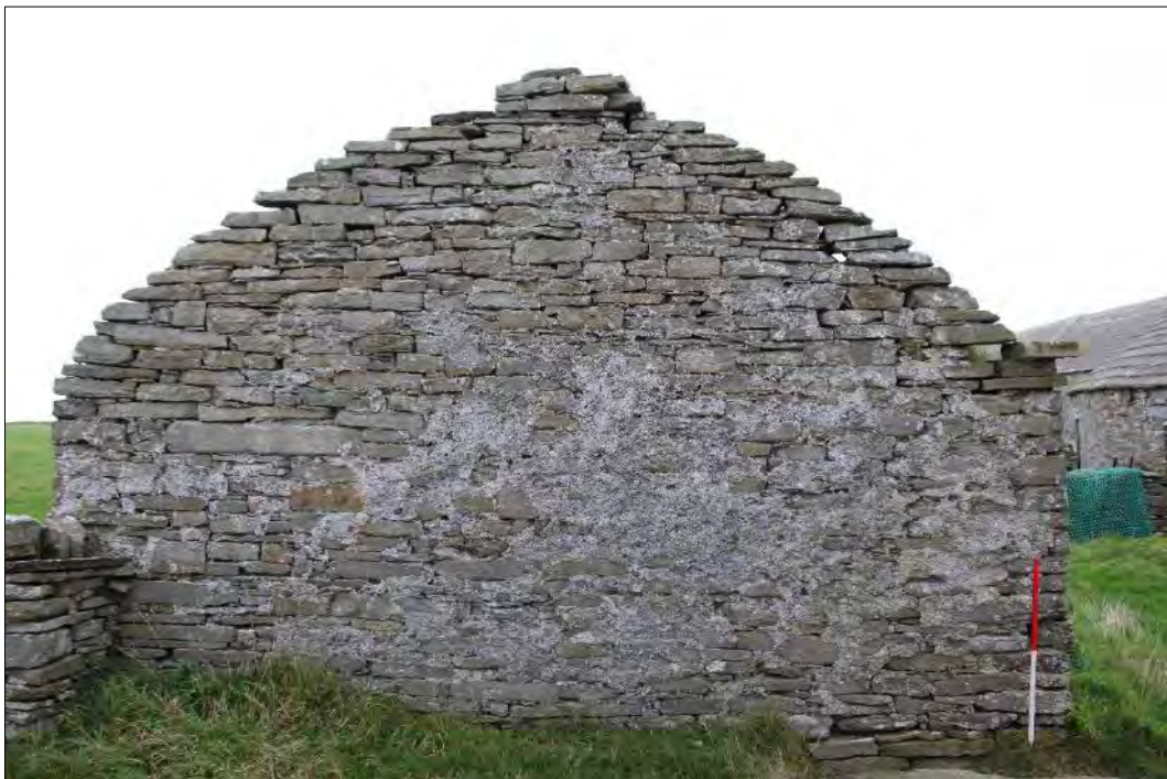
Plate 107: West-facing gable end of Building 13 illustrating the slightly convex nature of the gable. The blocked small window is visible towards the north end (left).
