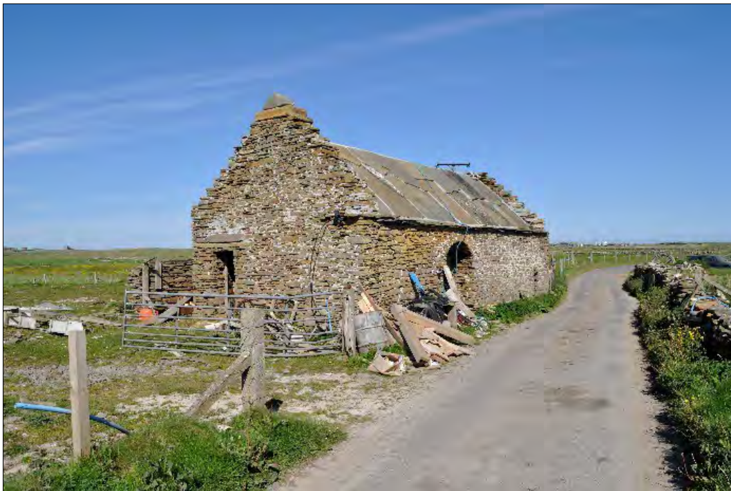
Plate 43: General view of Hooking Mill, looking east northeast (June 2016).
