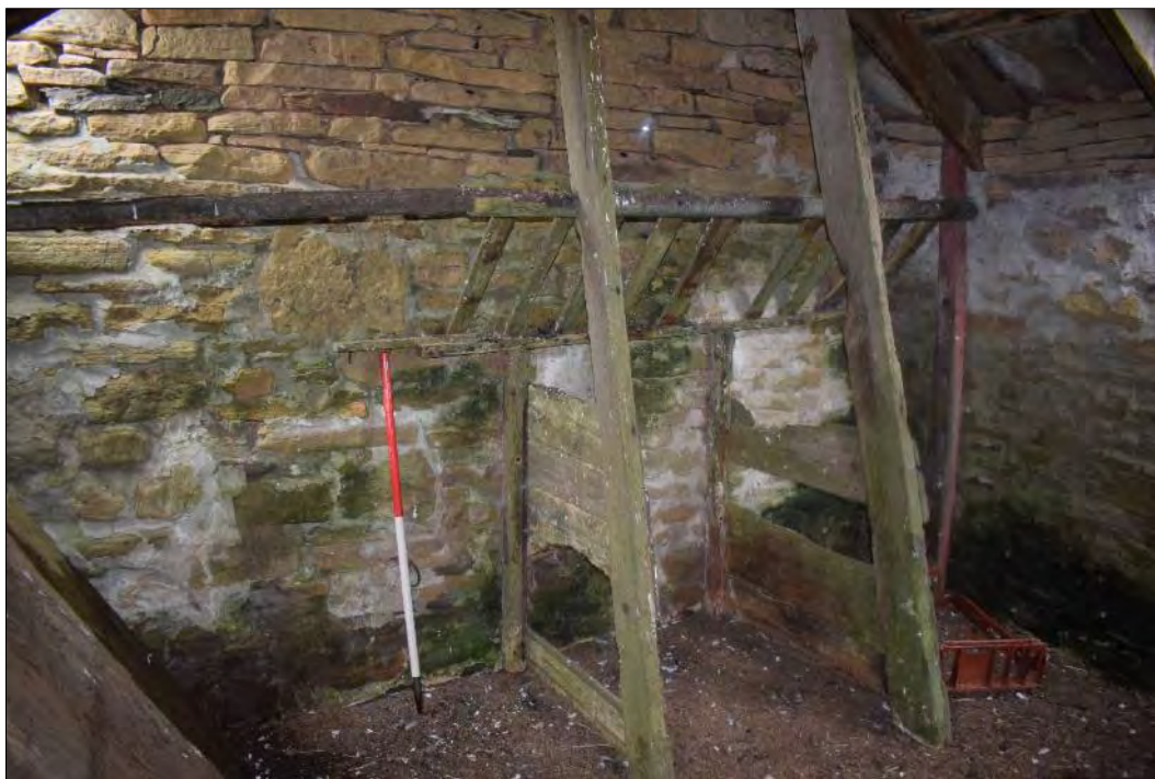
Plate 177: South elevation of Building 4, Quarryhouse, with two, in-situ timber-built animal stalls.
