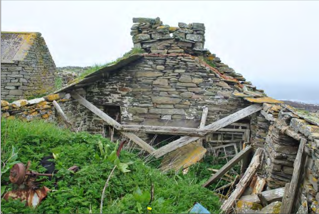
Plate 117: Northeast elevation of FB 4 showing fireplace, lumb, integral cupboard and remains of the flagstone roof.
