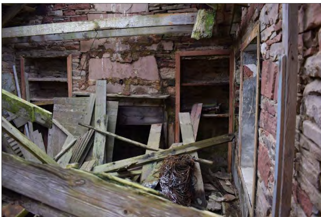
Plate 24: Building 2, east elevation with central fireplace flanked by integral cupboards.
