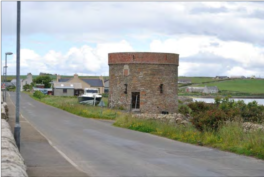
Plate 137: General view of the gasometer, looking northeast.
