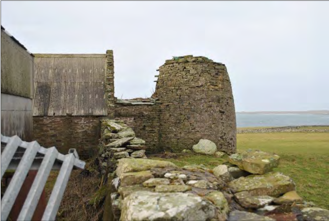
Plate 96: General view of the corn drying-kiln at the north end of the old threshing barn (Building 10), and linked by a short, roofed passage.
