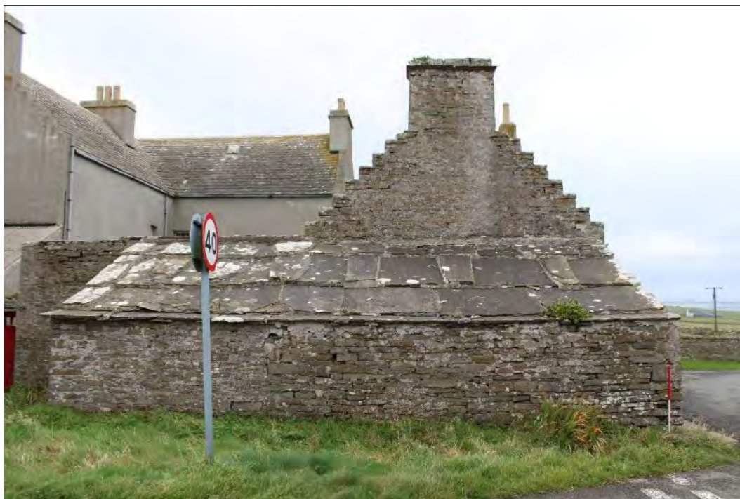
Plate 75: The north-facing elevation of Building 3.2 viewed from School Road showing how the wall extends beyond the gable end reflecting the original plan of the structure. Much of the elevation is obscured by a lean-to structure (Building 3.3).
