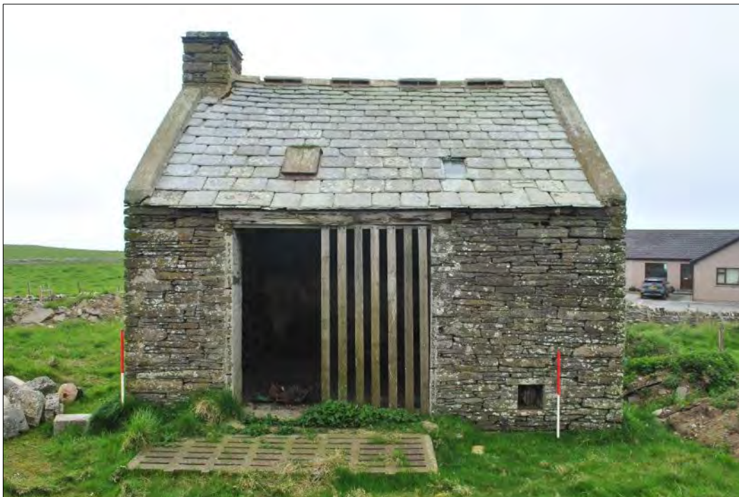
Plate 130: North-facing elevation of the slaughterhouse showing large doorway and ventilation hole.
