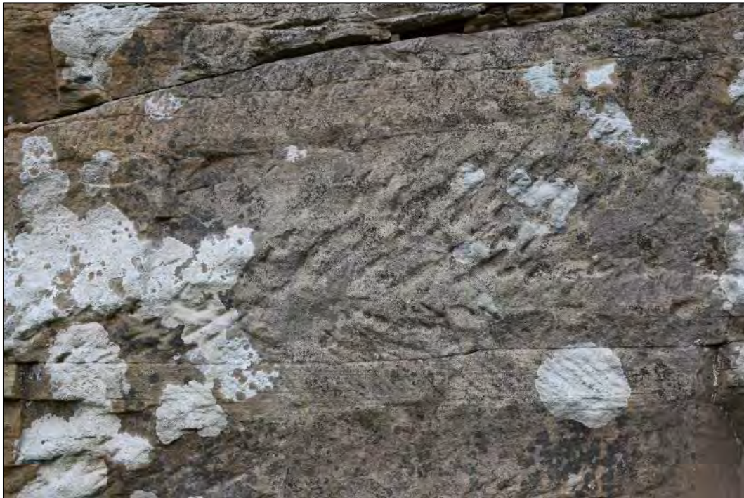
Plate 171: An example of the tooling marks visible on the working faces.
