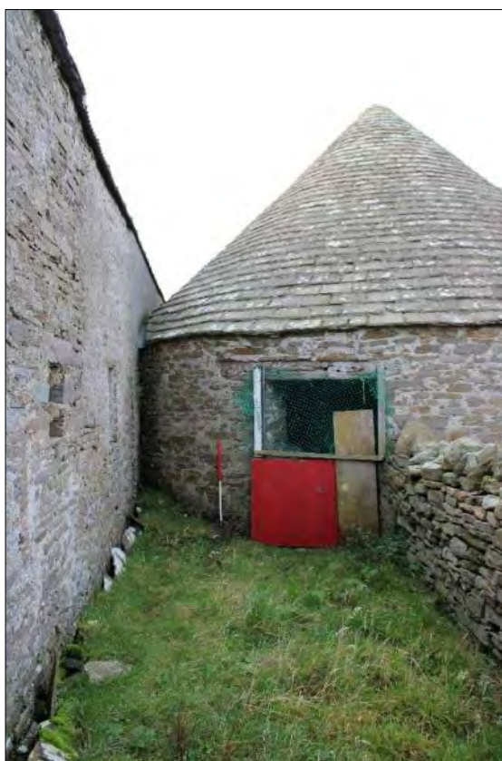
Plate 12: The horse-mill at Holland, Papa Westray. The building is circular in plan and the horse would circumambulate the interior to power the mill. This particular example provided the power for a large threshing machine house in the building to the left.
