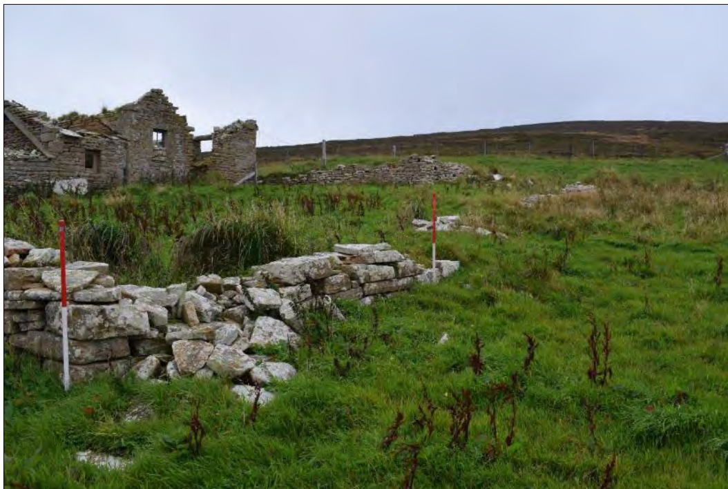
Plate 179: General view, looking southeast, towards the northwest corner of the enclosure wall (Structure 8) showing the curvi-linear form of the north-south wall at its north end – a relict form preserving the line of the roofed, boat-shaped structure which originally stood at this corner of the enclosure.
