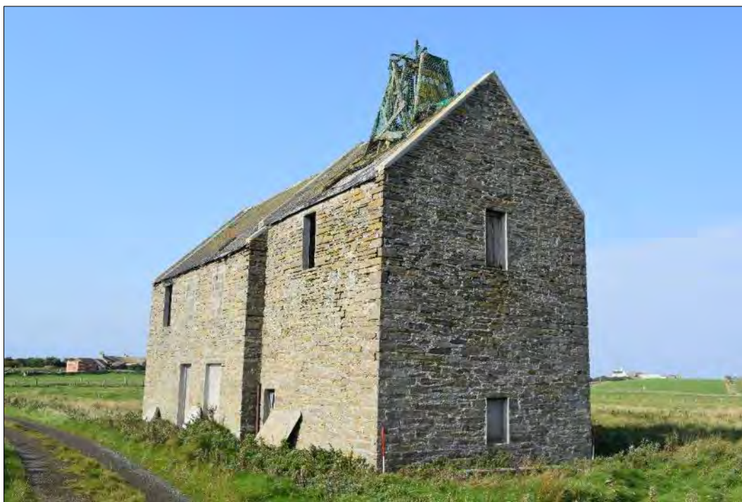
Plate 10: The engine-powered mill at Millhouse, North Ronaldsay. The corn drying-kiln occupies the northeast end of the building, closest to the camera. The timber structure protruding through the roof is the kin vent which allows the escape of the hot air rising from the kiln. Others examples seen across the North Isles, such as Meikle Mill, possess more modest kiln vents.
