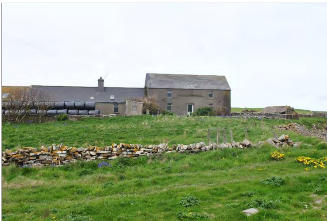
Plate 119: South-facing elevation of FB 5 (right centre) and FB 6. The chimney stack in FB 6 probably marks the division between the centre and west (left) structure shown on the First Edition 25-inch OS map.
