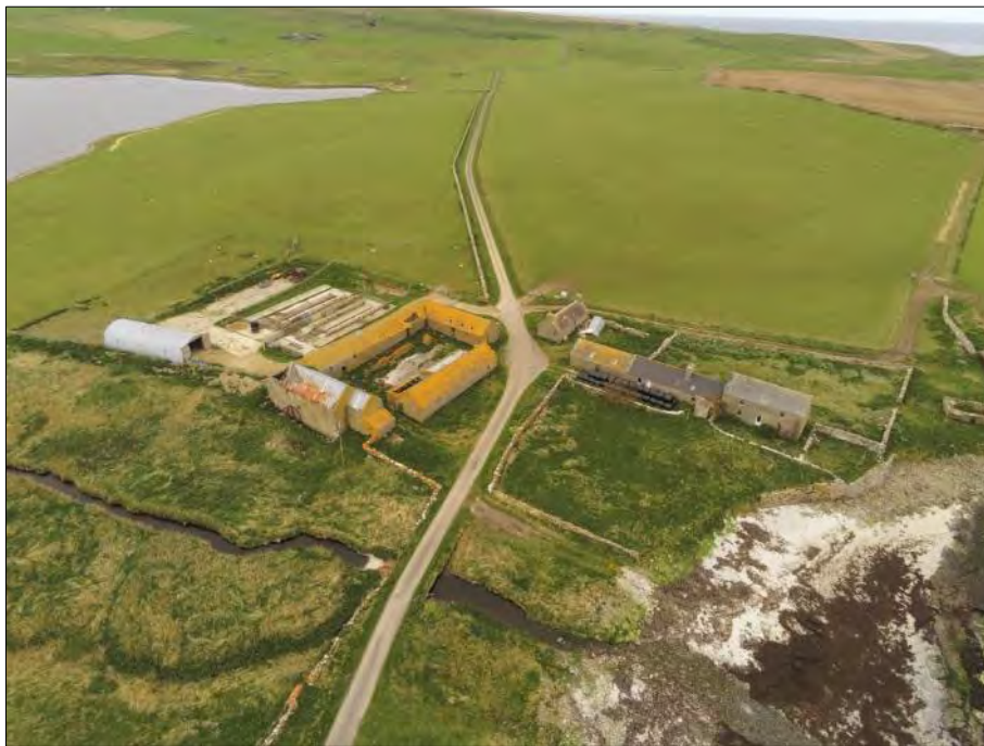
Plate 118: Aerial view of Saviskail Farm, looking northwest, showing the domestic range (FB 5, 6, 7) and the single dwelling (FB 8) to the east of the road (right). To the west of the road are the free-standing byre (FB 9) and the complex containing the water-powered mill (FB 10) and the attached byres (FB 11, 12) (© Robert Friel).
