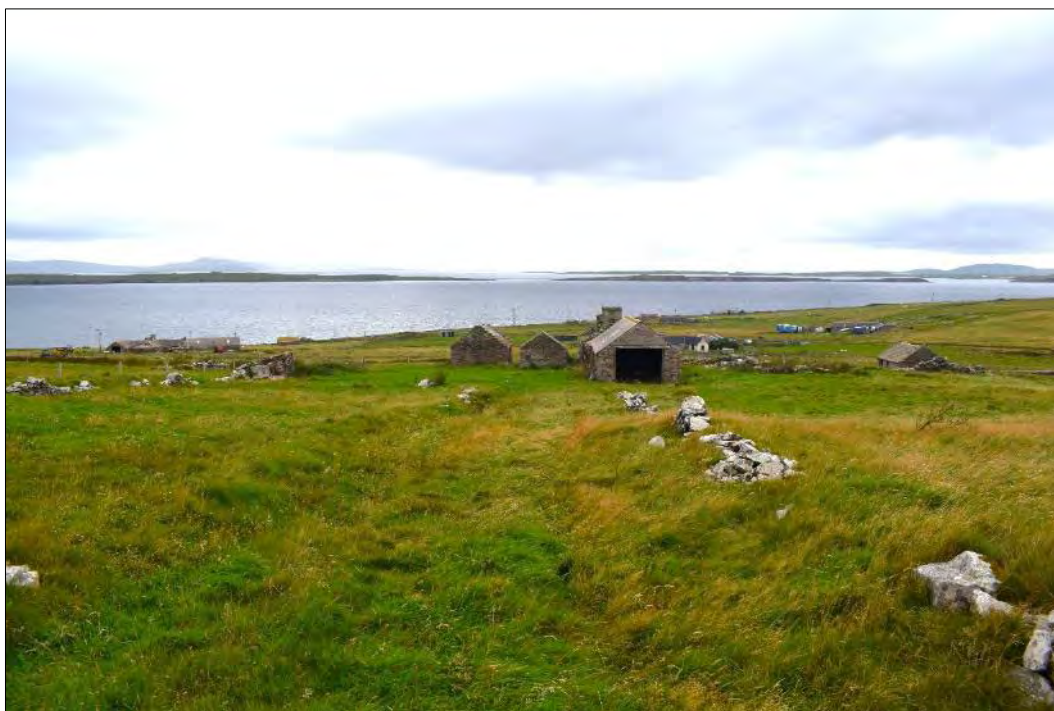
Plate 20: General view of Redhouse looking west towards the Sound of Faray. The view shows the three ranges comprising the main farmstead complex along with remains of enclosure walls (foreground)
