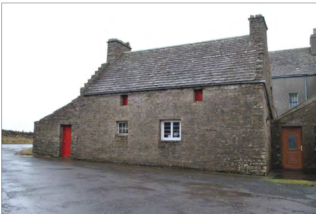
Plate 73: General view of Building 3.2 looking northeast from Central Road. The construction scar below the left ground-floor window is clearly visible, as is the construction break between this structure and the lean-to (Building 3.3) at the north end. The lean-to structure on the right with the modern door butts against the south wing and service wing of Holland House (Building 3.1)
