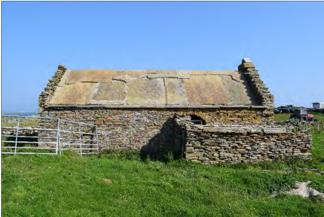
Plate 45: Southwest-facing elevation of Hooking Mill showing the later lean-to structure.
