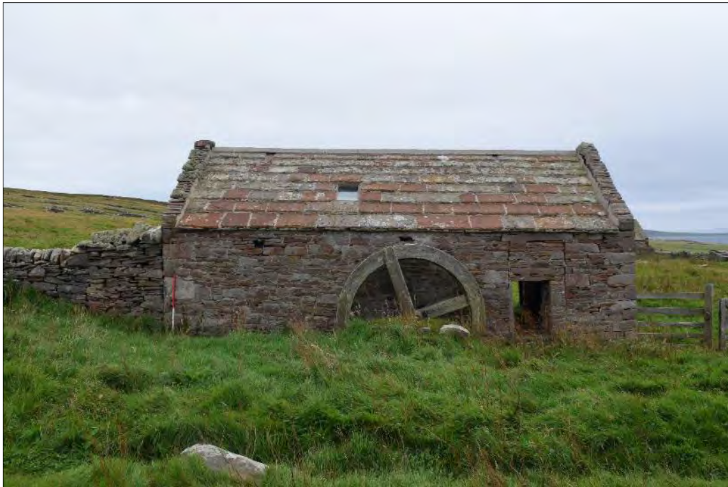
Plate 40: General view of Building 17, looking south, showing the mill-wheel and the modified external doorway.
