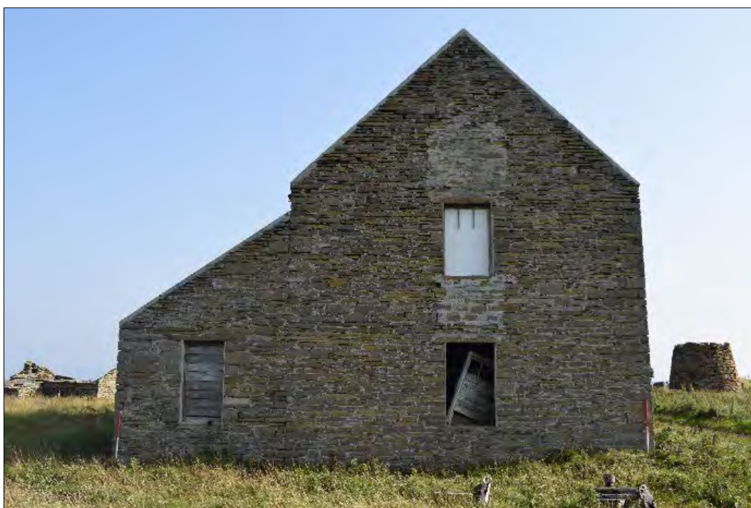
Plate 50: Southwest-facing elevation of the later mill showing the lean-to structure housing the engine (left).
