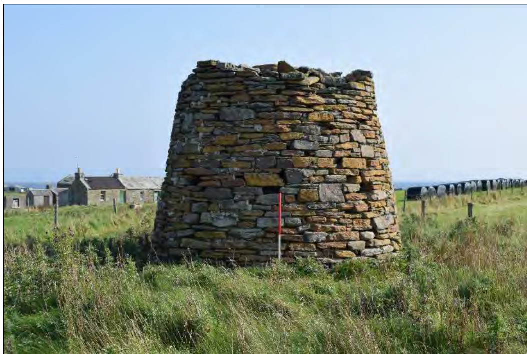
Plate 11: The windmill base at Millhouse, North Ronaldsay. This is an example of a turret post mill which would be topped by the timber-built main body of the windmill sitting on a timber post supported by the stone-built base. A drawing from c.1908 shows that this windmill had a long tail beam which allowed the main body to be revolved thus turning it into the wind.
