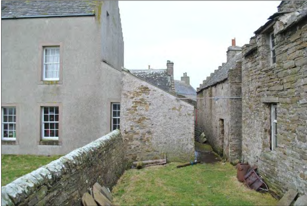
Plate 65: View looking west at the rear of the buildings on the corner of Central Road and School Road. The largest is Holland House (left and centre) with the south-facing elevations of Building 2 (centre right) and Building 1 (right) visible.
