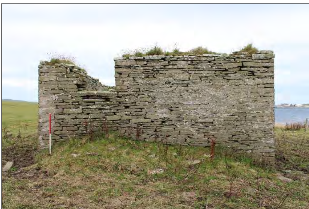
Plate 167: Southwest-facing elevation with truncated first-floor doorway.
