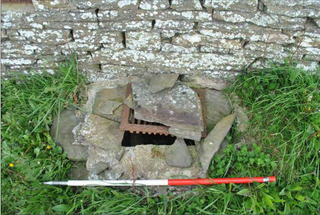
Plate 133: Detail of the south-facing elevation showing the drain head.
