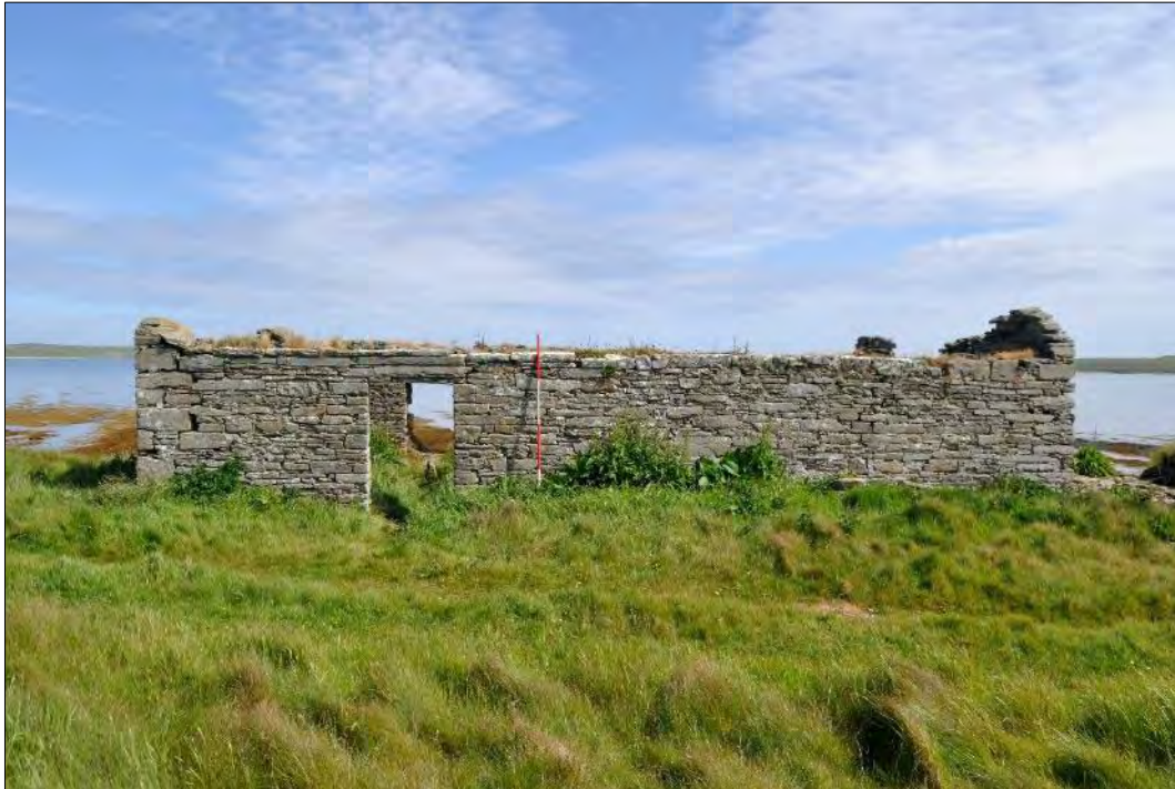
Plate 57: South-facing elevation of Hookin Mill, Papa Westray (June 2016).
