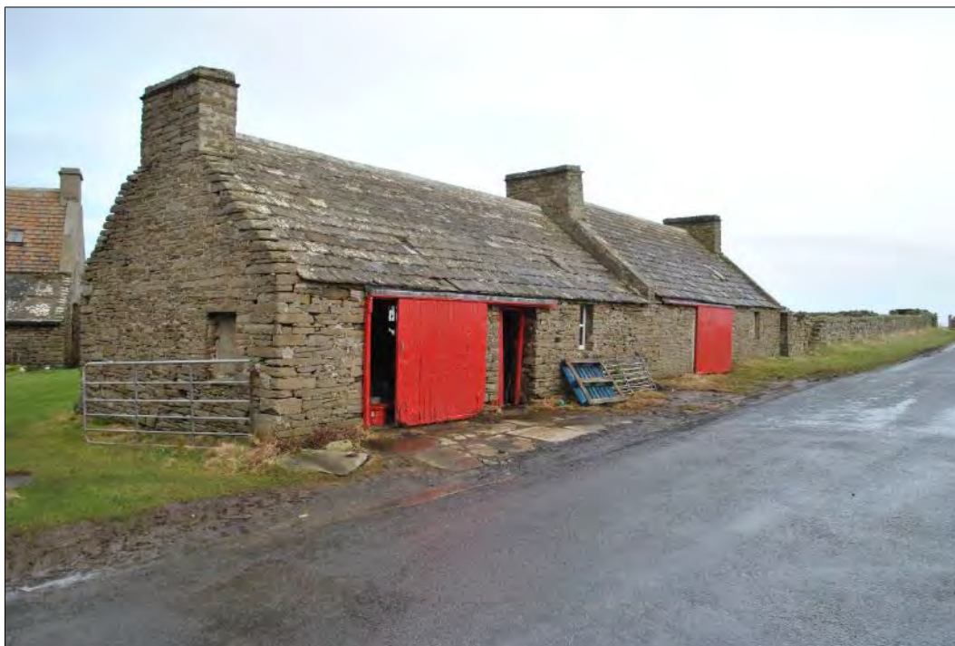
Plate 77: General view of Building 4 looking northwest from Central Road.
