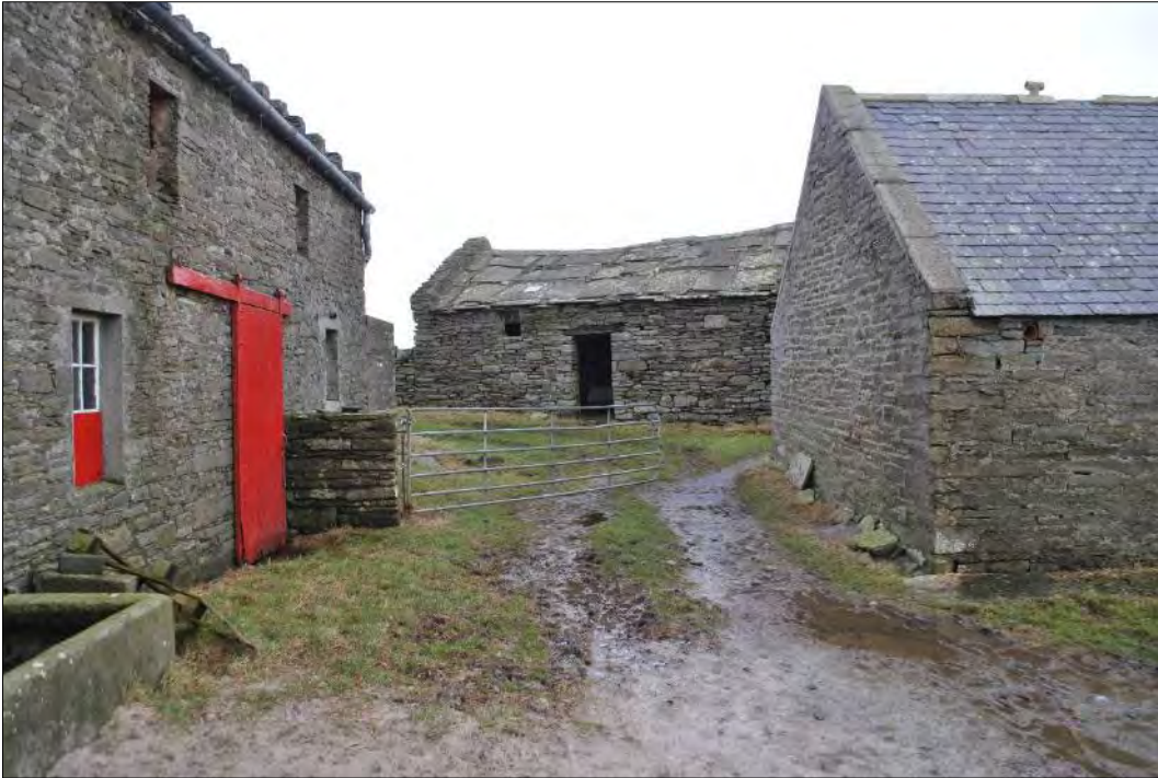
Plate 80: General view of Building 5, looking northeast, with Building 6 on the left and Building 8 on the right.
