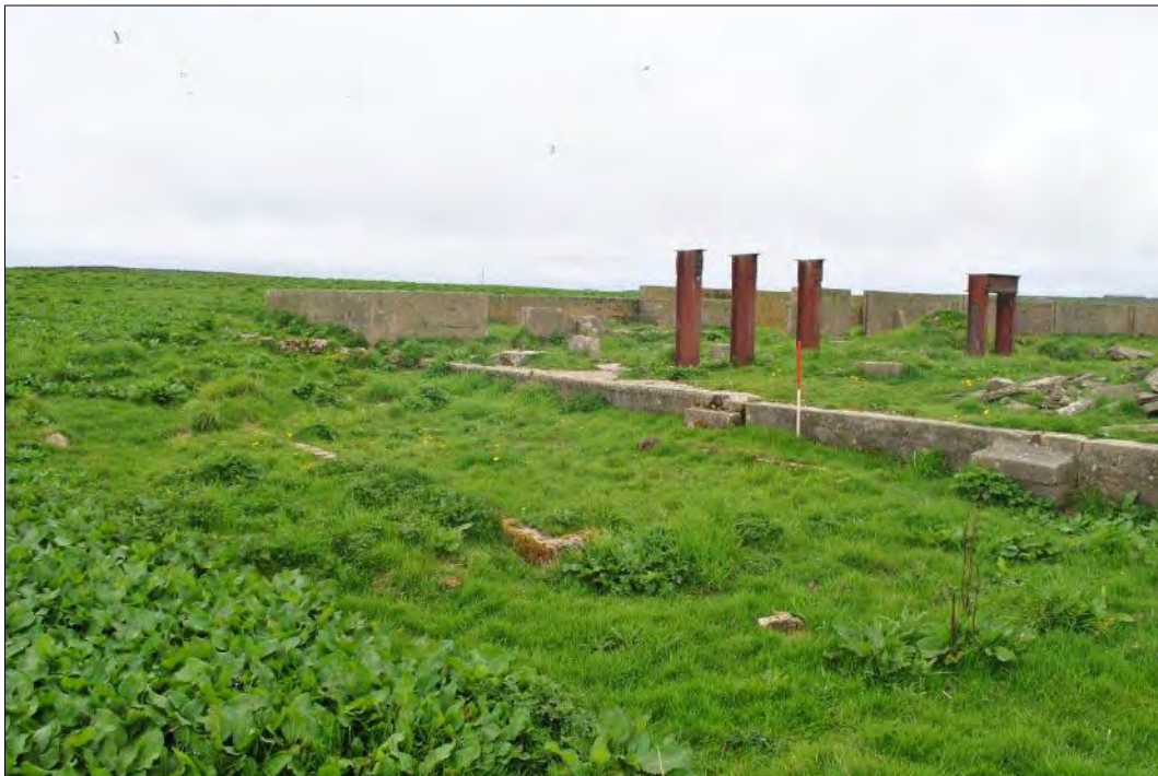
Plate 204: General view of the southeast edge of the plant showing the open-ended concrete structure outwith the raised platform area and the earth-fast concrete blocks partially obscured by vegetation.
