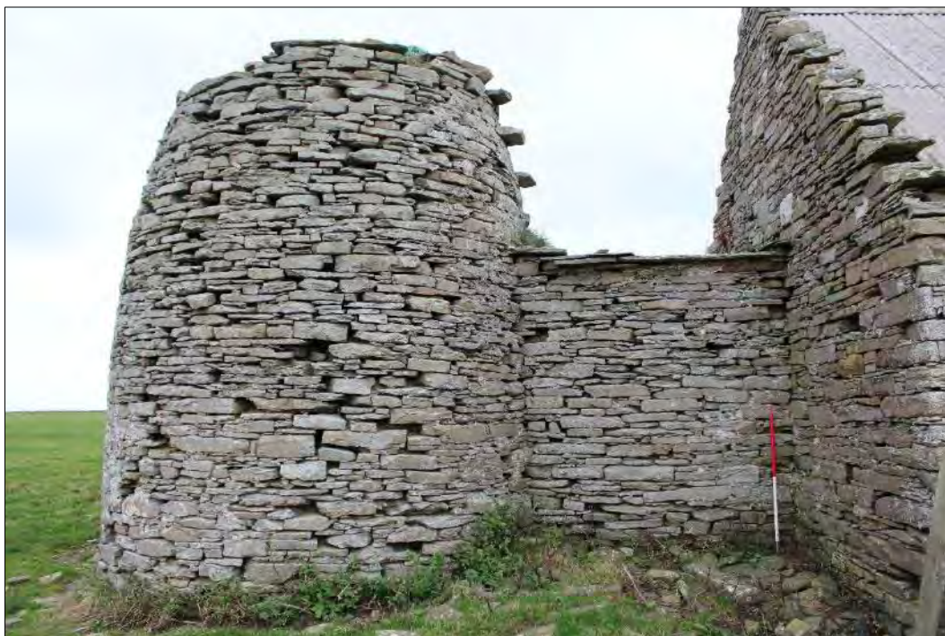
Plate 99: Detail of the corn drying-kiln (Building 10) showing the short linking passage with flagged roof and the outstanding stones forming a staircase leading to the top of the kiln.
