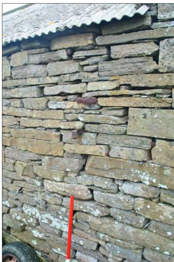
Plate 120: Shoe-last inserted into the stonework of FB 7, north-facing elevation.
