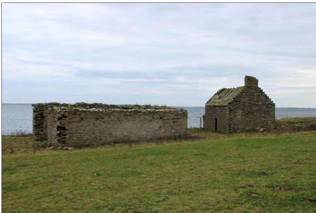
Plate 165: General view looking west towards the north building and the cornhouse.
