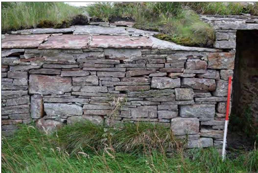
Plate 26: Detail of north-facing elevation showing construction break (extreme left) between Building 3 (centre and right) and Building 4.
