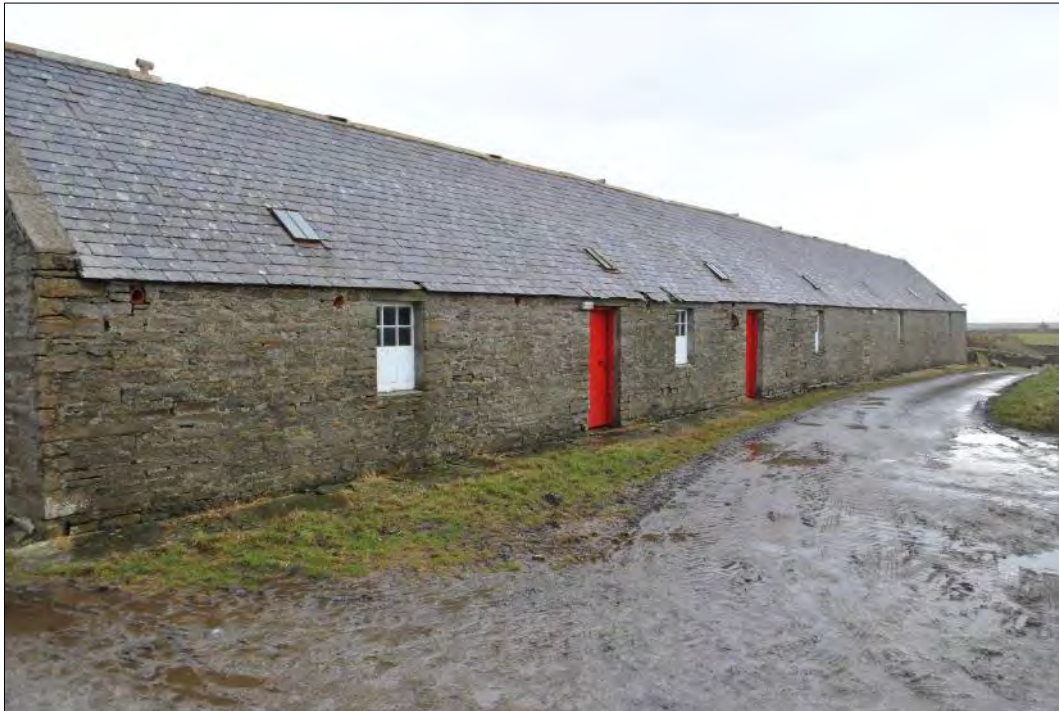
Plate 92: East-facing elevation of the cattle byre, Building 8, looking southeast.
