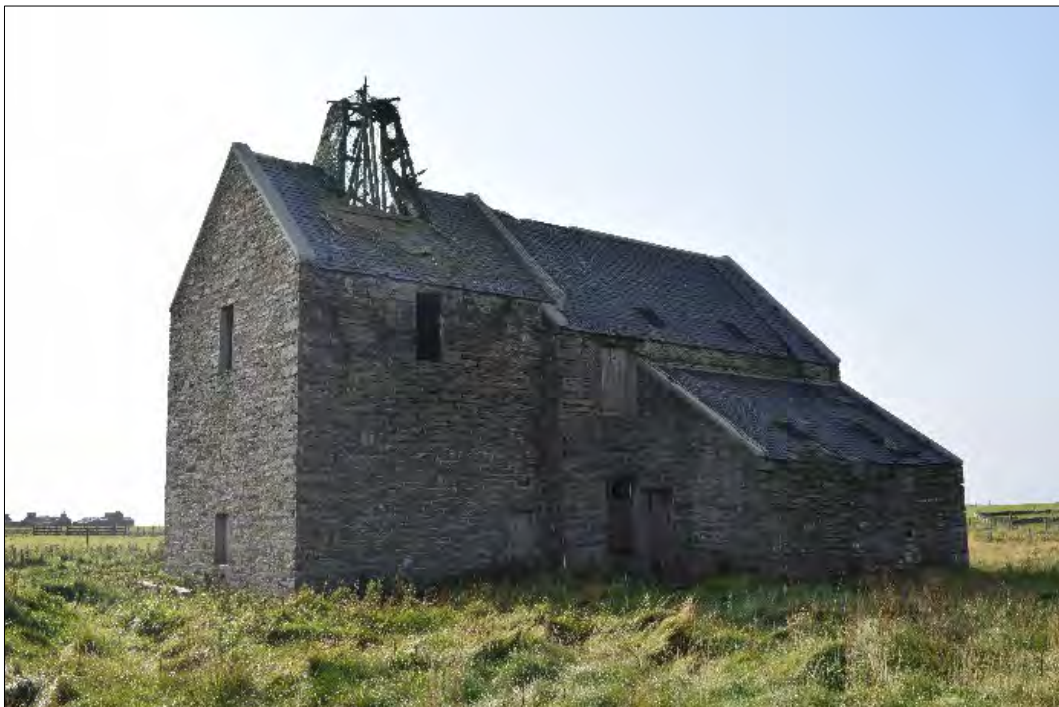
Plate 49: General view of the engine-powered mill, looking southwest, showing lean-to (right) and the large kiln vent in the roof towards the northeast end of the building.
