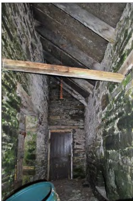
Plate 152: Corn-drying kiln - view along the passageway linking the front exterior doorway (centre) and the rear doorway (behind camera). The doorway on the left leads to the main ground floor room. The main kiln structure is on the right with the fire charging hole at the base.
