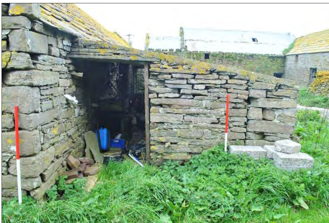
Plate 122: North-facing elevation of lean-to structure FB 9.1 showing external doorway and construction break which may indicate the structure was originally open-sided.
