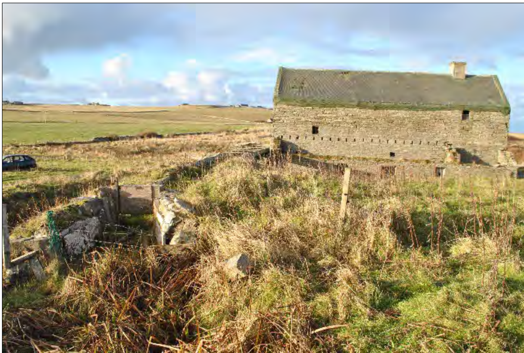
Plate 155: General view, looking northwest, showing the mill (right) with the stone-lined head race (left) leading to the timber trough and roofless wheel house (centre).
