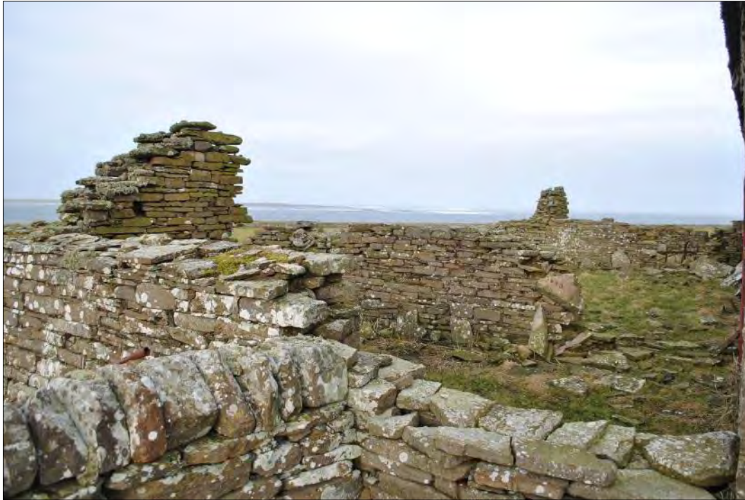
Plate 100: General view of the sheep sheds, Buildings 11 and 12, looking northwest from the southwest corner of the old threshing barn.
