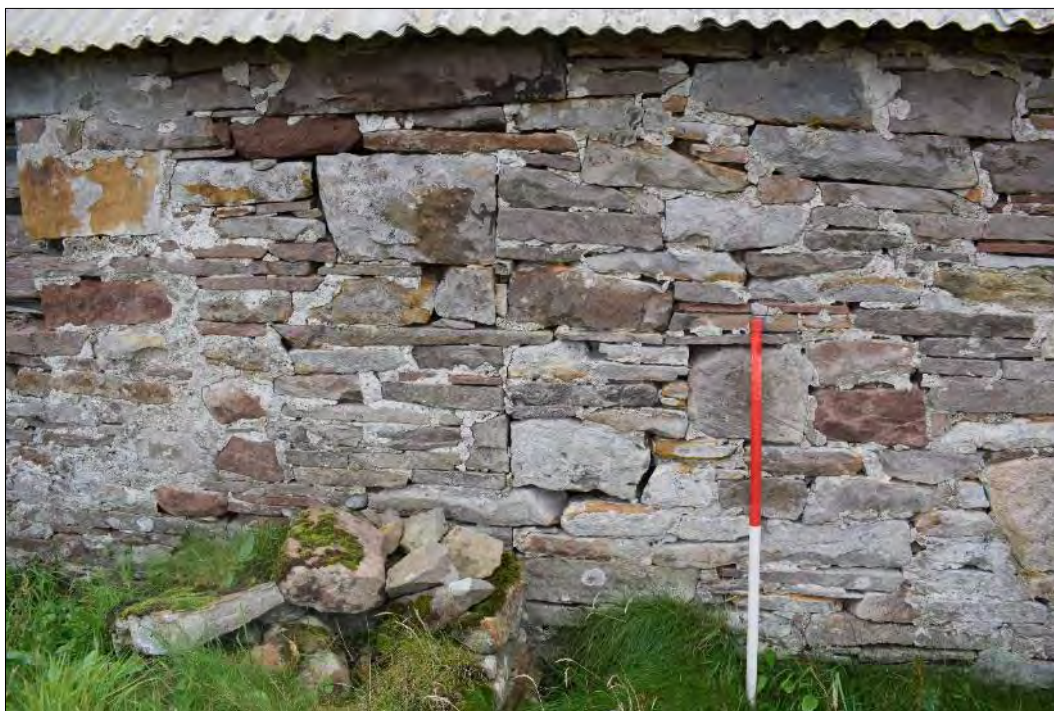
Plate 30: North-facing elevation showing the wall scarring which marks the former division between Building 5 and 6. The remains of the former enclosure wall at the base are keyed into the elevation.
