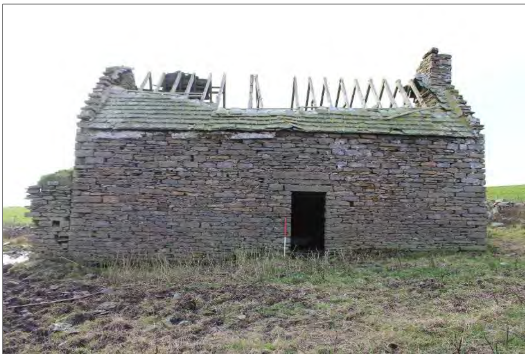
Plate 159: North-facing elevation of Cornhouse
