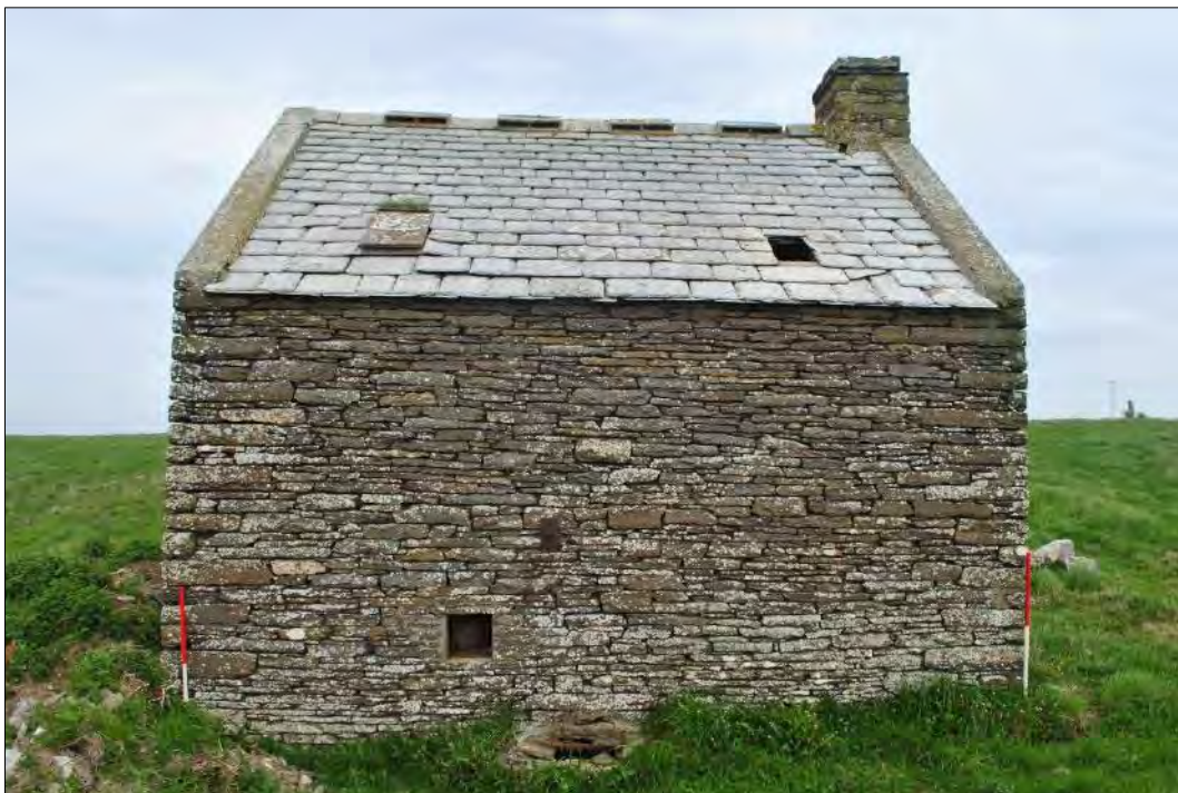
Plate 132: South-facing elevation of the slaughterhouse showing ventilation hole and drain head in the ground surface at the base of the elevation.
