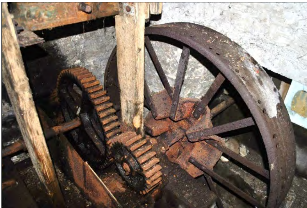
Plate 148: Mill machinery located on the ground floor. The shaft extending from the hub of the large wheel connects to the hub of the exterior water wheel.
