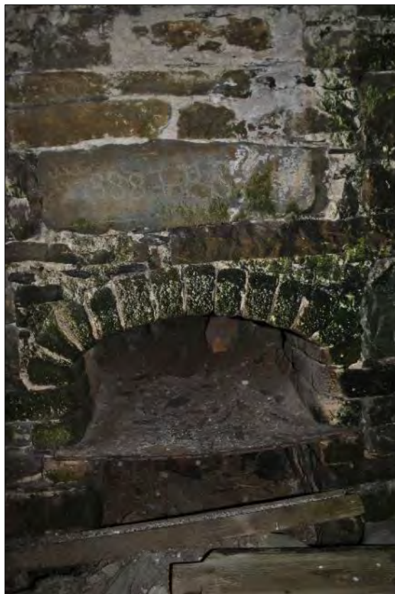
Plate 153: Detail of the kiln charging hole showing the iron grate and the graffiti above.
