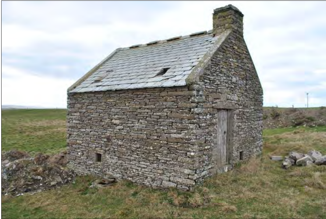
Plate 129: General view of the slaughterhouse, looking northwest.
