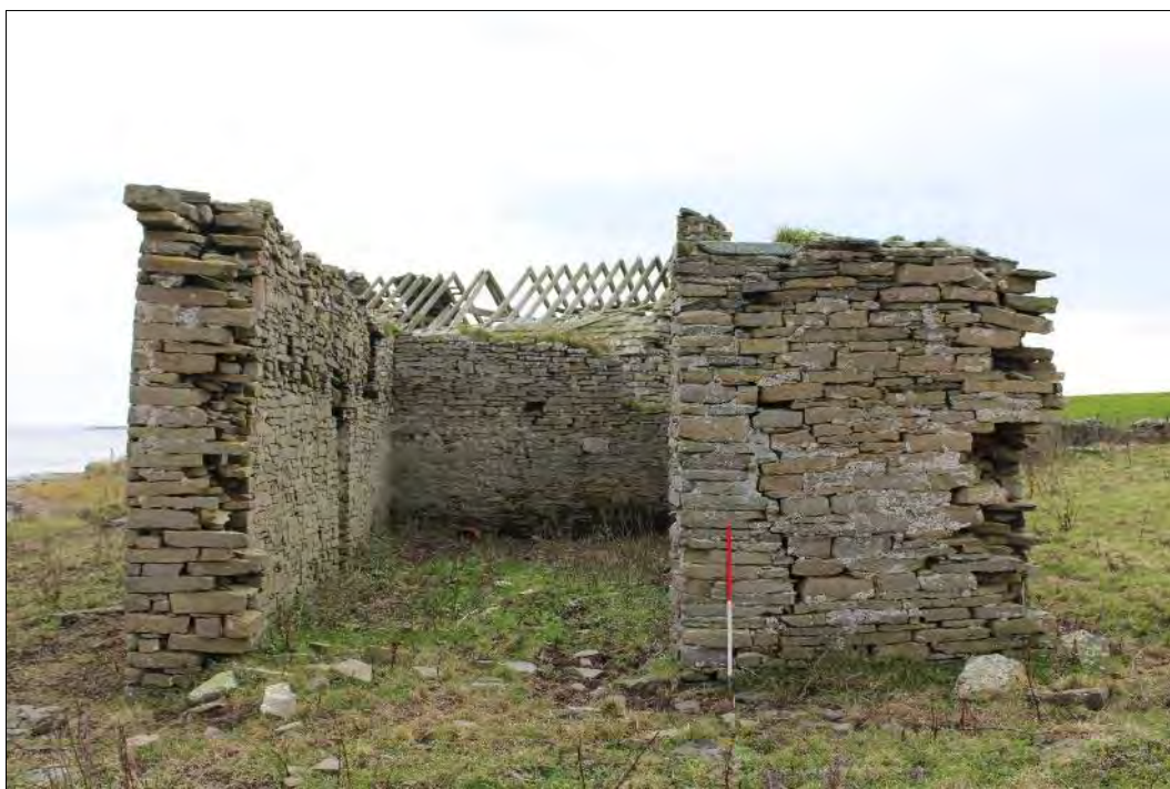
Plate 166: Northwest-facing elevation with large exterior doorway.
