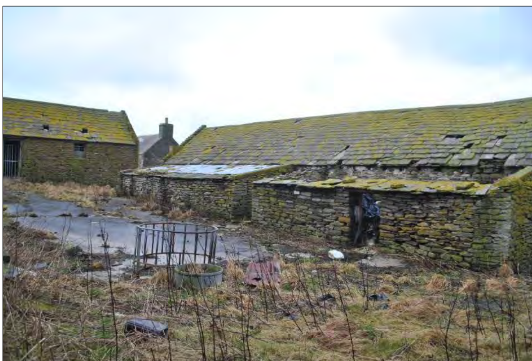
Plate 121: General view from the southwest corner of the quadrangle looking north towards FB 12 (left) and the lean-to structures built against the west-facing elevation of FB 9.
