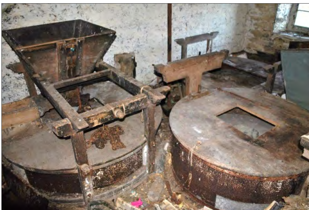
Plate 149: Two of the three grindstone pairs within their casings on the first floor of the mill building.
