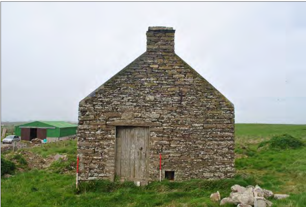
Plate 134: East-facing gable of the slaughterhouse showing the doorway, ventilation and chimney.
