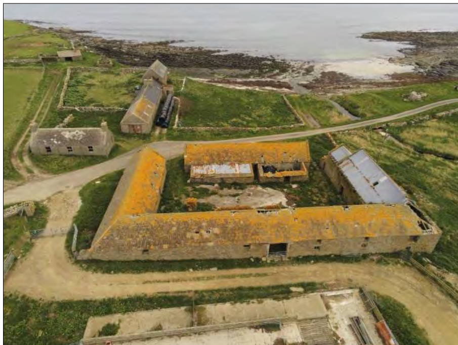
Plate 126: West-facing elevation of FB 11 illustrating how the sloping ground surface heightens the elevation and increasing the number of internal floor levels (© Robert Friel).
