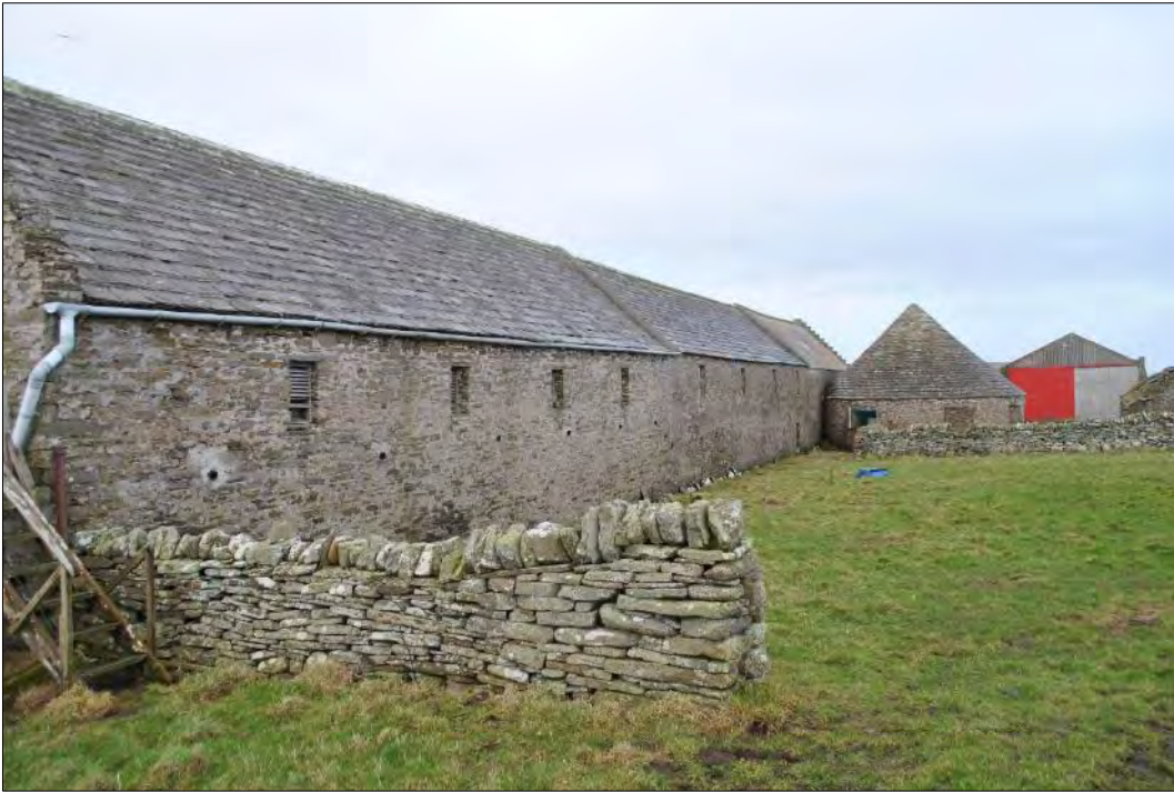
Plate 83: North-facing elevation of Building 6, with the stable (Building 6.1) nearest. The circular horse mill structure (Building 7) can be seen butting against the threshing mill (Building 6.3).
