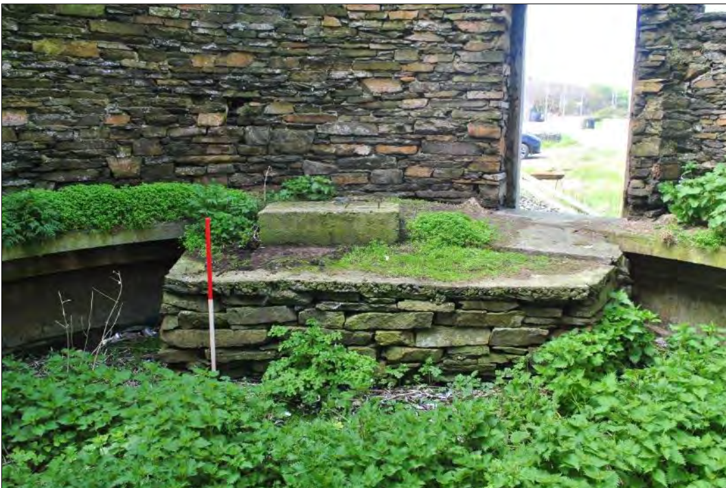
Plate 143: The stone-built platform within the circumference of the concrete ring, with a concrete base on its upper surface.
