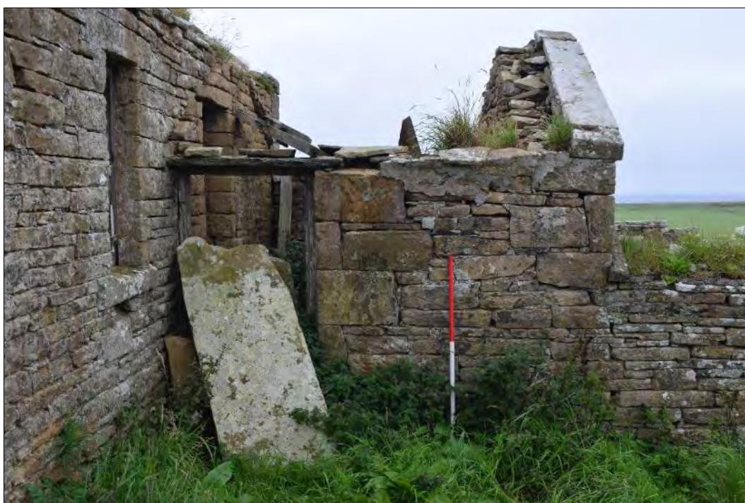
Plate 175: East-facing elevation of Building 2 at Quarryhouse showing external doorway and the exposed constituents of the north gable. The wall scar for the double pitched roof of Building 2 can be seen in the north-facing elevation of Building 1 (left) above the doorway of Building 2.
