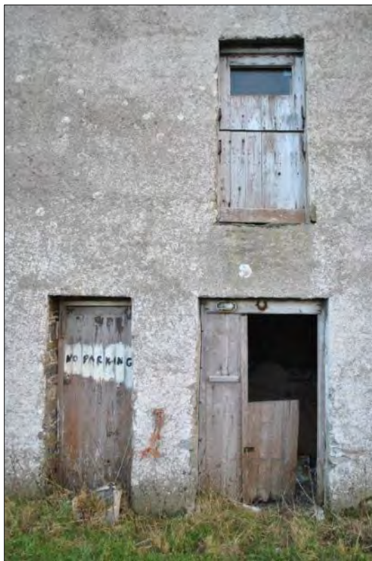
Plate 145: Detail of front (northwest-facing) elevation showing the ground floor main entrance (right) and the first floor doorway. The narrower ground floor doorway on the left provides access to the corn-drying kiln
