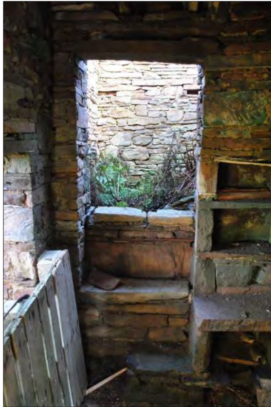
Plate 28: Corn drying-kiln, Building 4, looking north, showing the steps leading to the kiln floor and the fire hole (bottom right).
