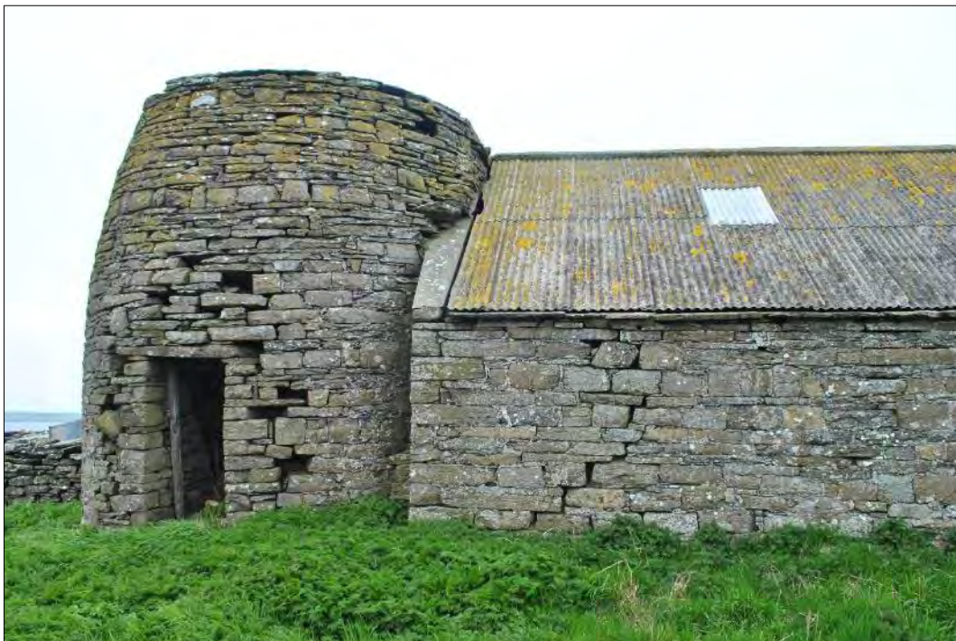
Plate 8: An example of a corn drying-kiln which formed an integral part of a farm building, usually a barn, which served a larger farm. This example is at Odin-ness, Stronsay and shows the typical bee-hive shape of the kiln's outer structure. The exterior access is unusual as the kiln floor and fire hole were more typically accessed via the interior of any attached building
