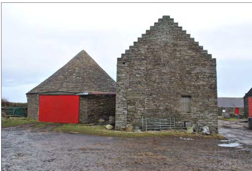
Plate 91: General view, looking northeast, showing the horse mill, Building 7 (left) alongside the threshing mill.
