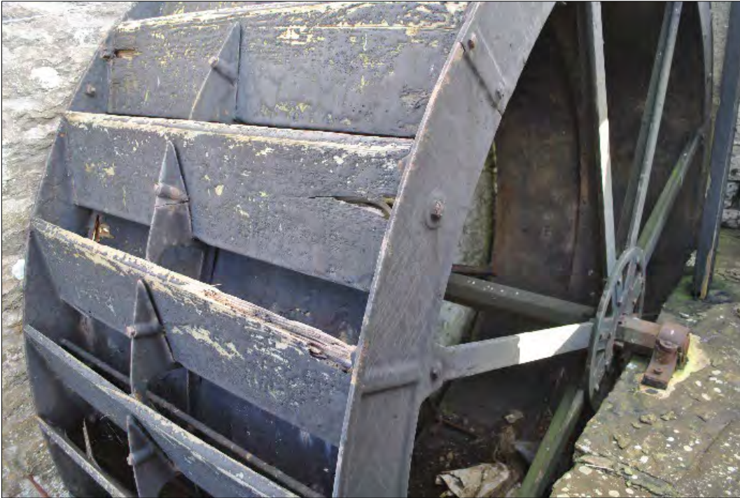
Plate 157: View of the water wheel, looking east, showing the axle seated upon masonry of the wheel pit, arms, rim and the buckets.
