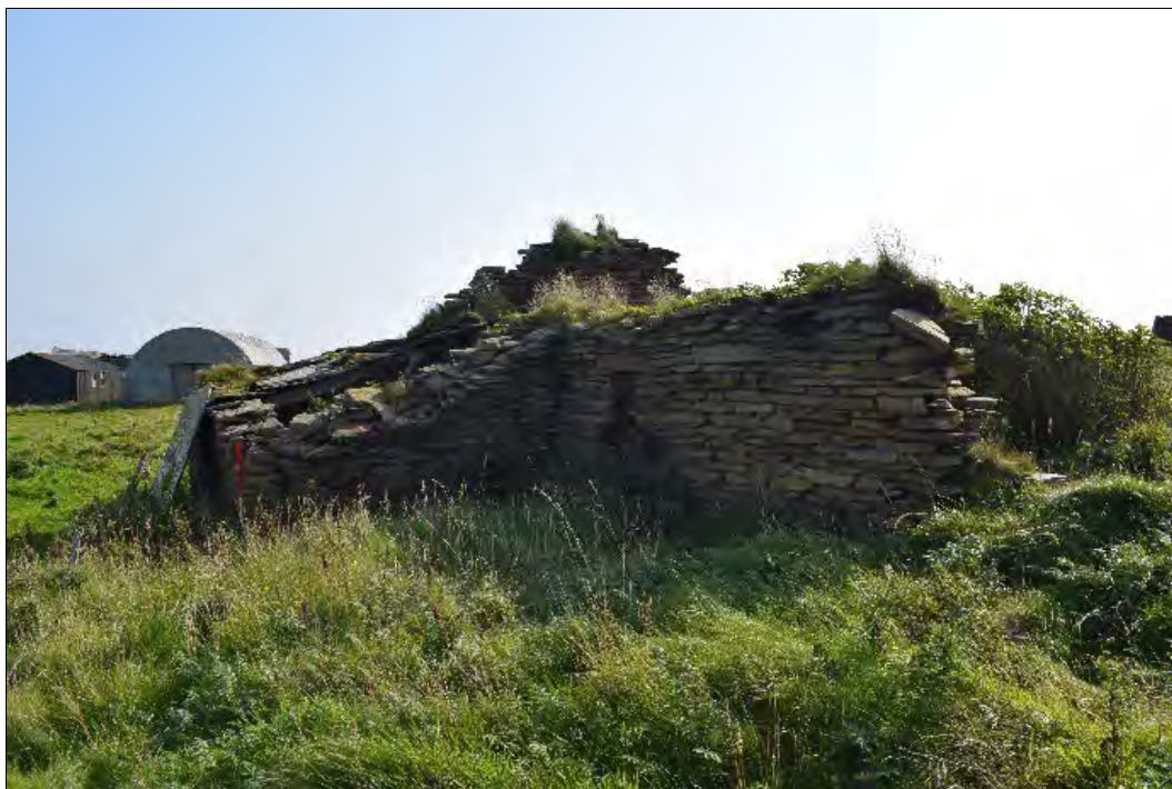
Plate 56: North-facing elevation of Millhouse, looking southeast, showing blocked doorway (centre) and the largely intact northeast annex.
