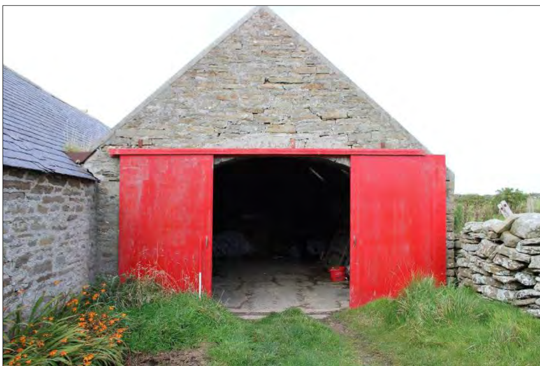
Plate 94: South facing elevation of the turnip shed, Building 9, with the segmented arch above the doorway visible behind the sliding doors.
