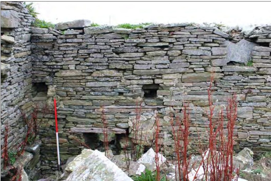
Plate 61: South elevation of Hookin Mill with one aperture at the base of the wall, a possible window (top right) and two beam slots (centre and centre left).
