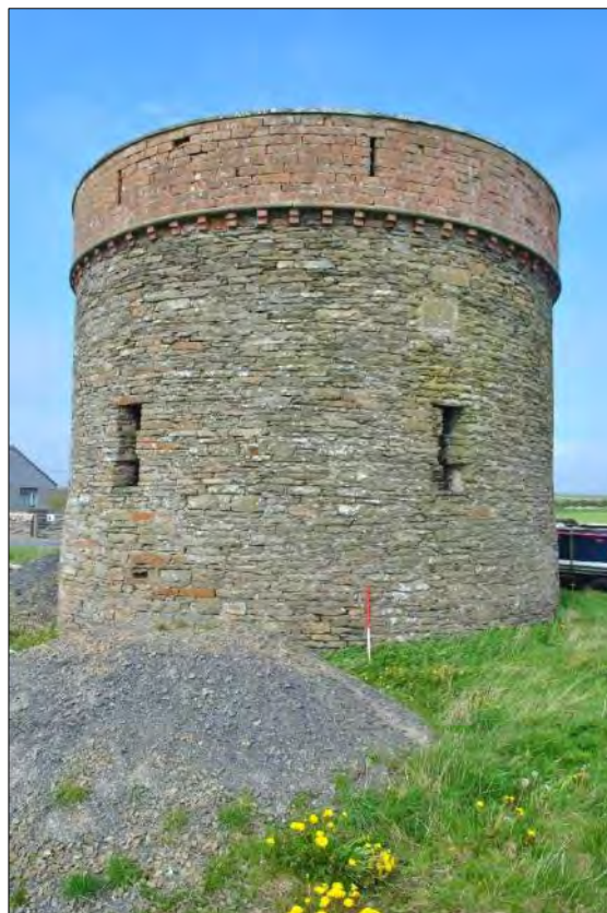
Plate 138: The gasometer, looking west, showing the red brick cap upon the stone rubble body.
